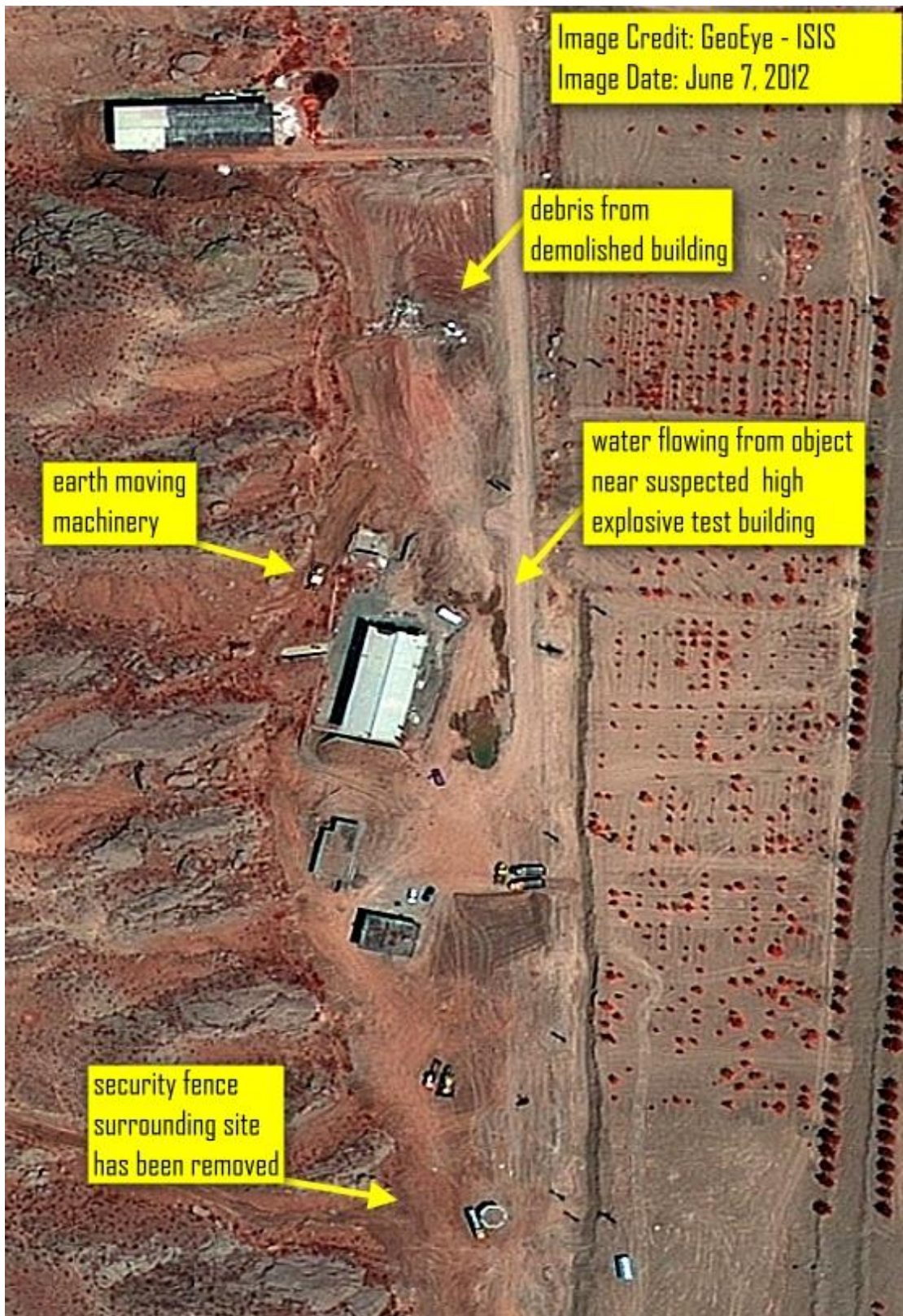
Figure 3: Imagery from June 7, 2012 shows the Parchin site at the height of the demolition and earth displacement process. The debris from the demolished buildings is visible at the site, the security perimeter has been removed, and there are heavy signs of earth displacement activity.
