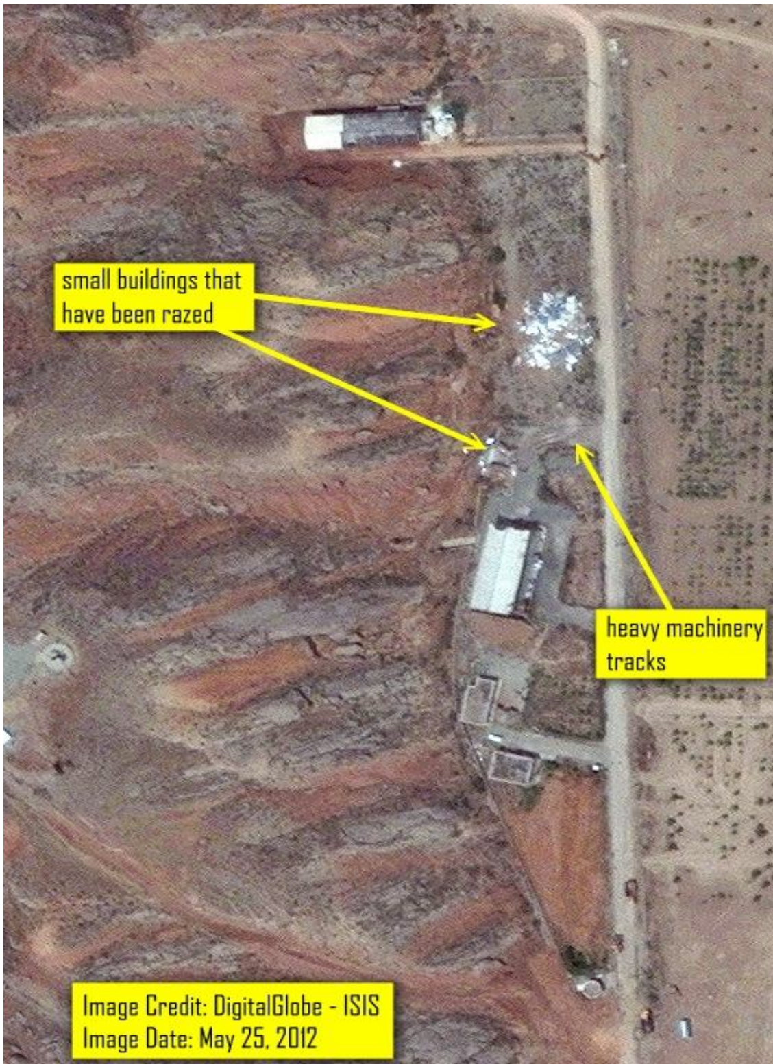
Figure 2. Earlier imagery from May 25, 2012 showing demolished buildings near the suspected high explosive testing building.
