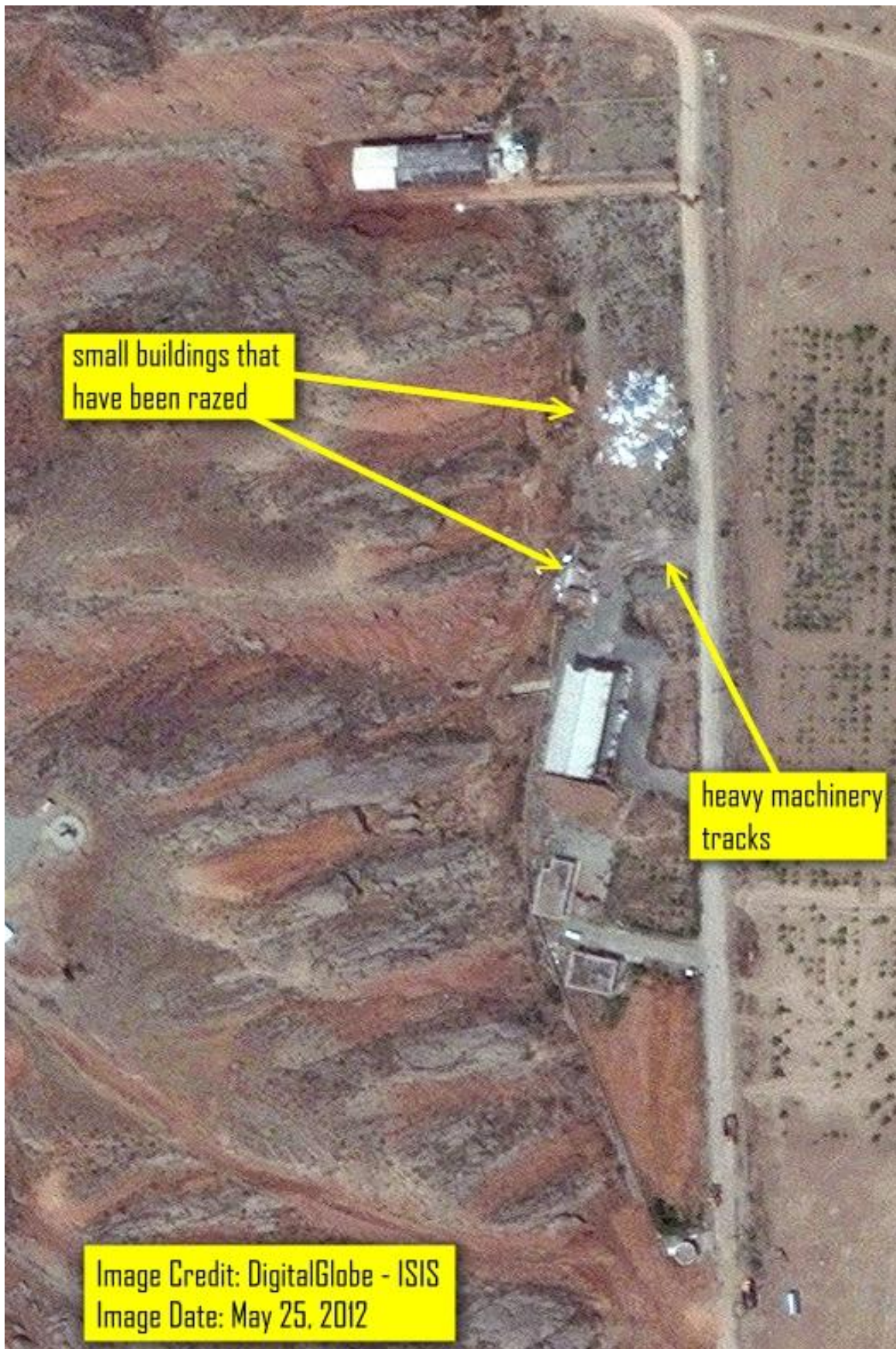
Figure 2. Imagery from May 25, 2012 showing the debris from the demolition of two support buildings located near the building suspected to contain the high explosive test chamber.
